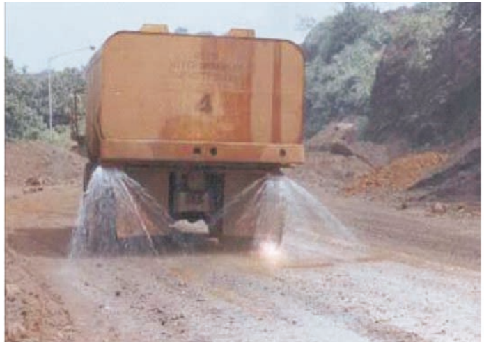
Water Sprinkling on Road for Dust Suppression
